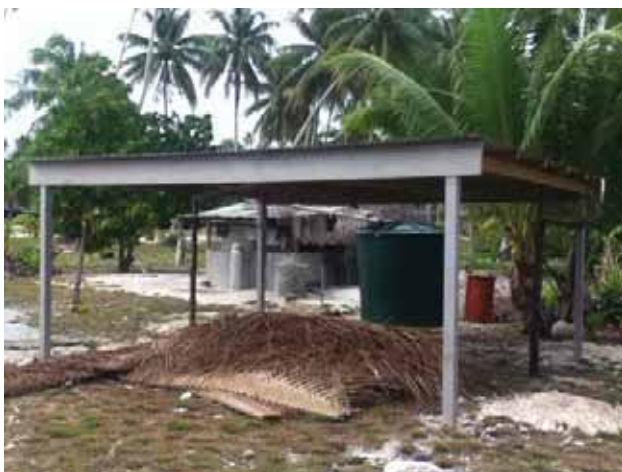
Traditional thatched houses on Nassau now with newly installed roof catchment, spouting and water tanks
