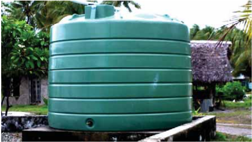
Existing 25,000L Aqua tanks that need repair
