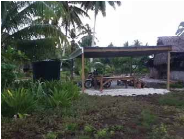
Traditional thatched houses on Nassau now with newly installed roof catchment, spouting and water tanks
