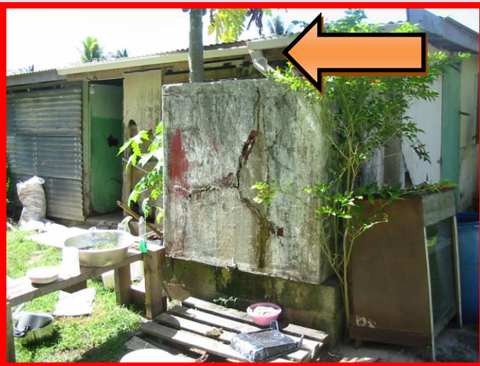
Photo: Some households repair old concrete box water tanks to increase their water storage capacity using materials that are affordable to them. Here is a classic case of downpiping falling away from the house structure. During the assessment this was seen on many homes in Atiu and Aitutaki.
