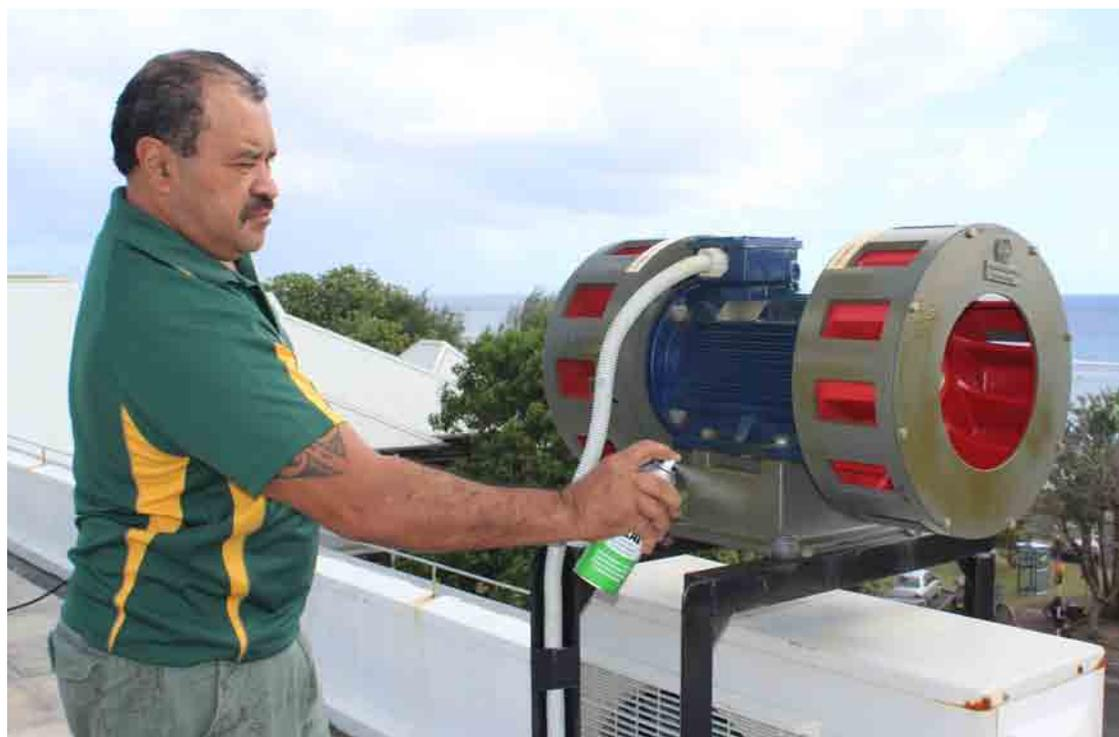
Charles Carlson applies anti-corrosion spray to the cyclone warning siren on the police station roof in Rarotonga
