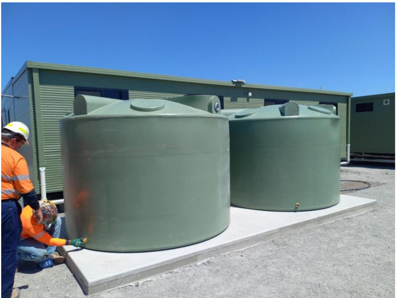
Figure 36 Water Tank installation
