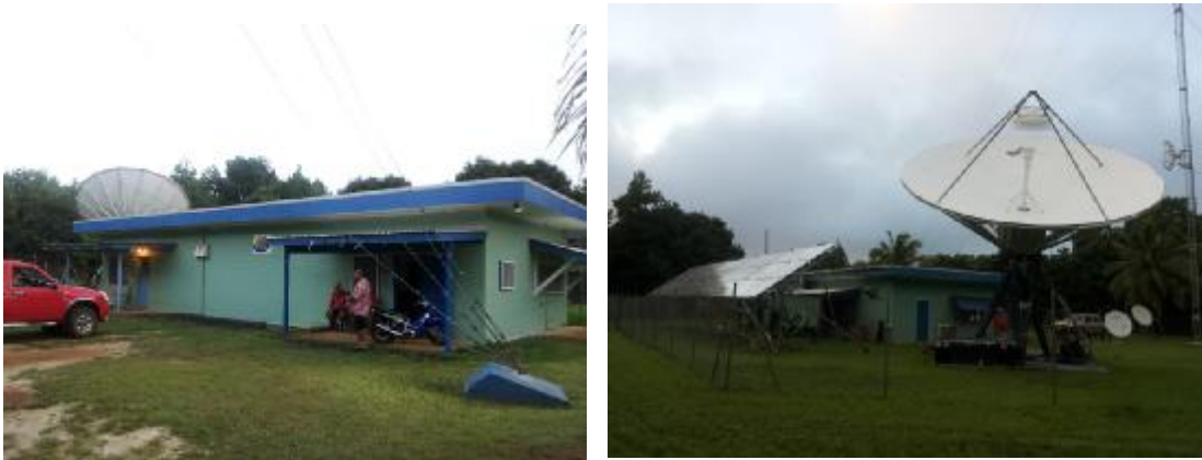
Figure 9: Atiu Telecom Station that also has the Atiu Radio station
